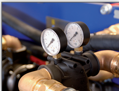
Process water system integrated into the machine sub-frame
